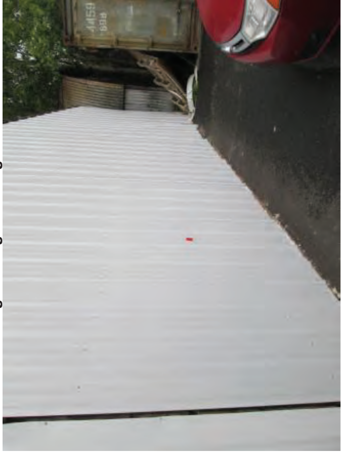
A-3. Old Bldg. South Side Looking East
